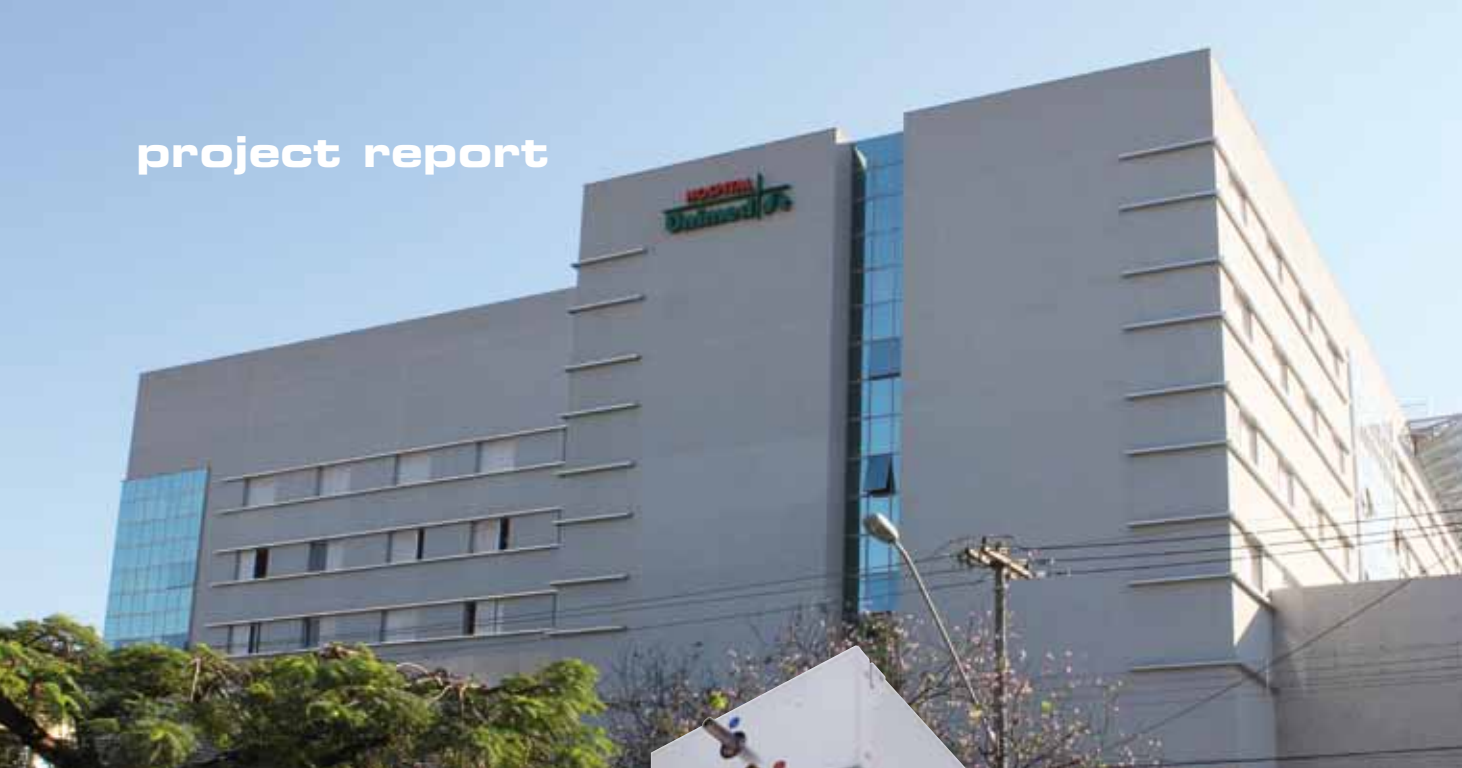
Santa Bárbara, Brazil Hospital Unimed de Belo Horizonte
