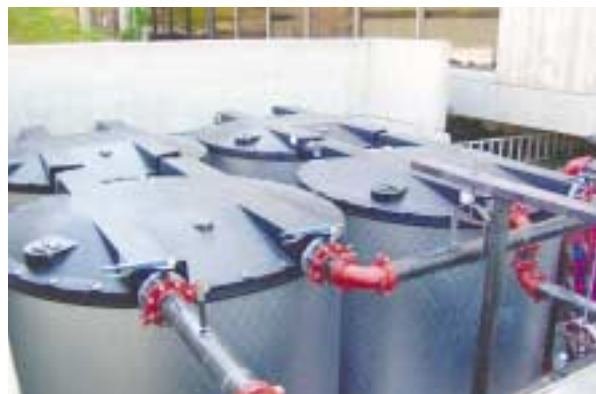
Two Model 1320C tanks being installed
