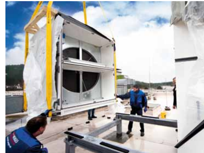
Roof installation on prepared steel structure
