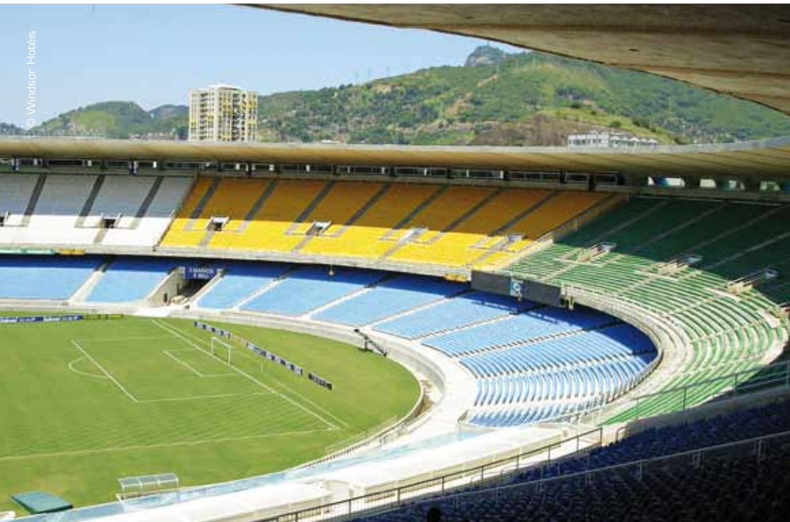
Behind the listed façade, the time-honoured Maracanã Stadium ...
